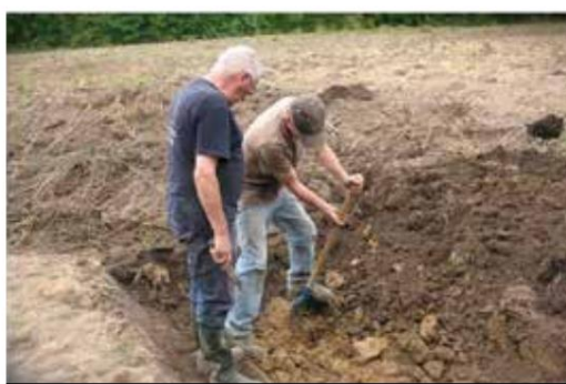
A real work of digging
